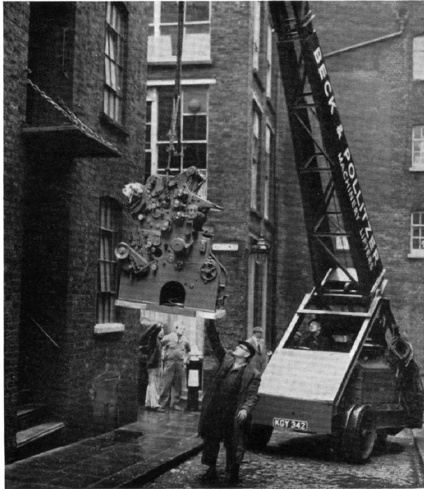
New plant arriving at our Hutton Street factory. It looks easy, but there was over two tons of complicated machinery at
